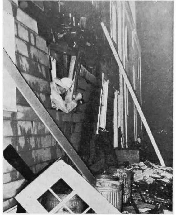
The blast that bulged the walls blew out windows, doors and pieces of the ceiling. Third floor sleeping quarters miraculously were undamaged.
