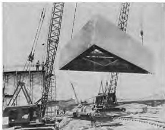
Construction equipment swinging portion of arch structure into place under Brother Kolkmeier's direction.
